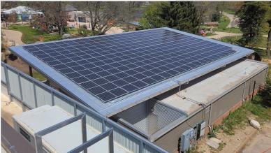
with ample sunlight, these panels can generate up to 70 amps per phase, which is then fed back into the main distribution panel.
